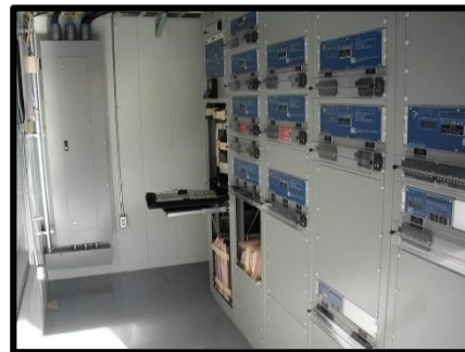
Protective Relays in Substation
