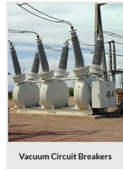
Figure 1.10: SF6 and Vacuum CB
