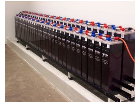
DC Supply System in Substation
